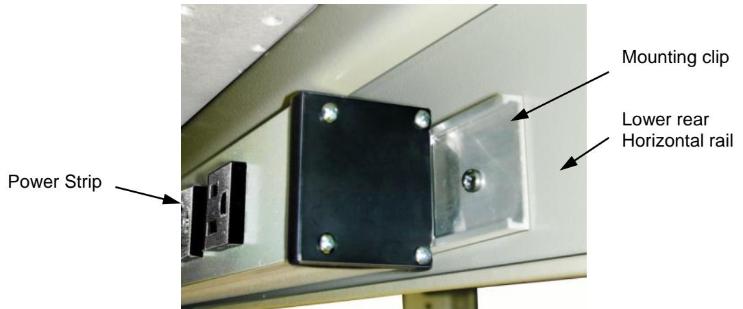
Figure 23, Power strip installation
